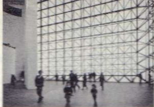
Cover: The John Fitzgerald Kennedy Library Columbia Point on Dorchester Bay, Boston, Massachusetts Architects: I. M. Pei & Partners Photographer: Nathaniel Lieberman
