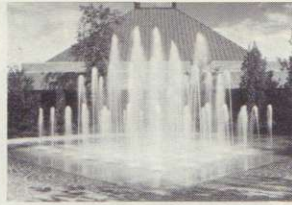
Cover: Administration and visitors center, Botanic Garden of the Chicago Horticultural Society, Glencoe, Illinois. Architect: Edward Larrabee Barnes. Photographer: ©Nick Wheeler
